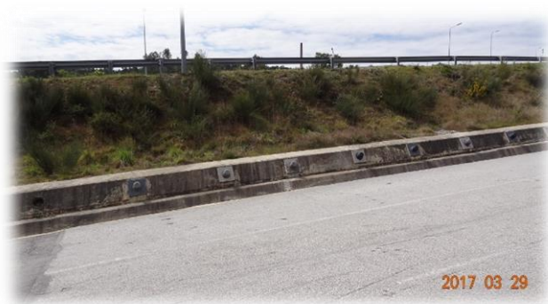
Anchored retaining beam and anchor pressure gauge.
