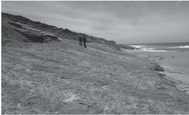
Fig. 2 – Landslide failure in Salgados beach.
