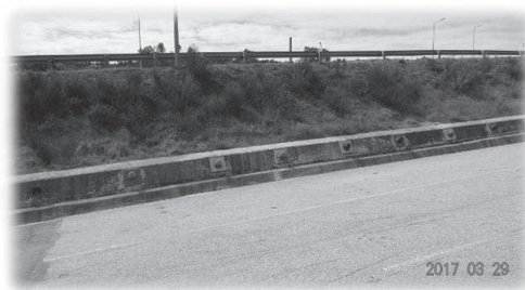
Anchored retaining beam and anchor pressure gauge.
